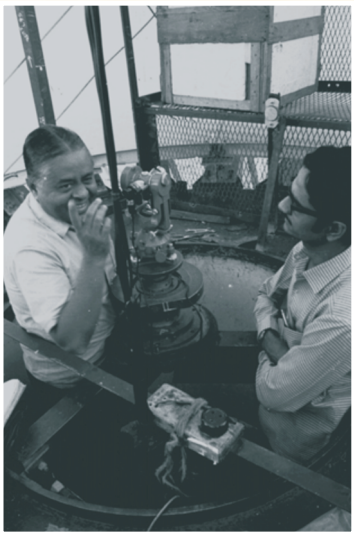
At the ARVI Antenna installation site Shri Ramaswamy, a expert in antenna alignment shares a lighter moment with Shri N.C. Bhavsar
